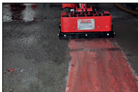
REMOVAL OF ANTI SKID COATINGS
