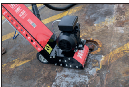
COATING & CORROSION REMOVAL
