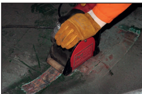
HAZARDOUS PAINT REMOVAL
