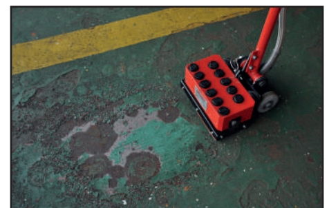
DUST FREE DESCALING
