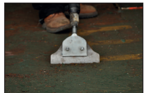
SHIP DECK RUST REMOVAL
