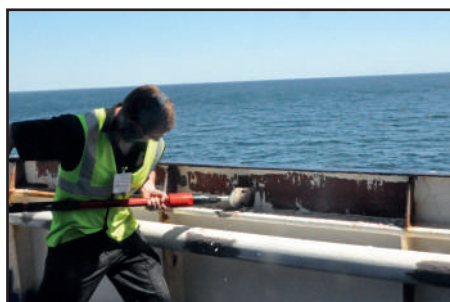
CLEANING STEELWORK
